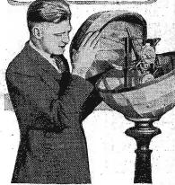
The heart of WJY-WJZ, an oscillograph that shows the Radie waves as they leave the antenna. This allows corrections to regulate the modulation, etc. There is an actual "motion" picture of the wave on the revolving square mirror. Operator W. E. Tesch is observing
